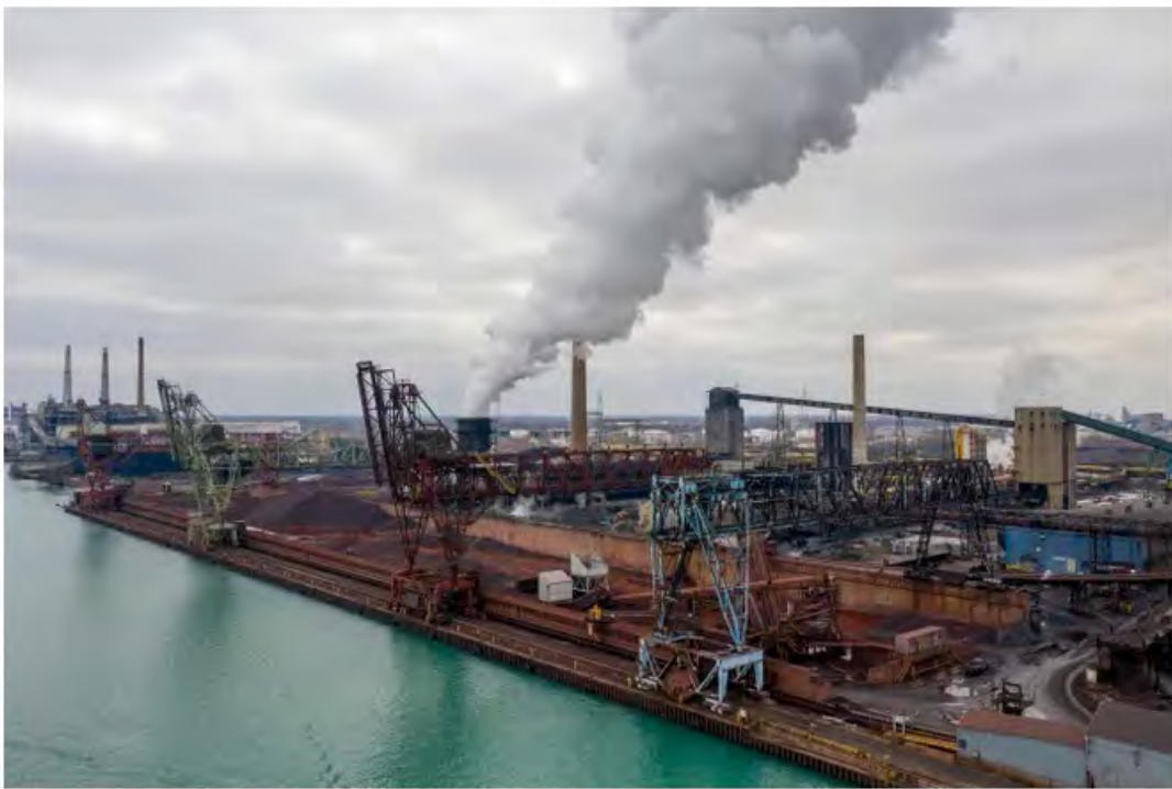
The EES Coke quenching tower erupts with steam as water is dumped on hot coke fresh from the ovens on a typical Zug Island day. The coke battery, once part of National Steel, is now owned by DTE. David Guralnick, The Detroit News
