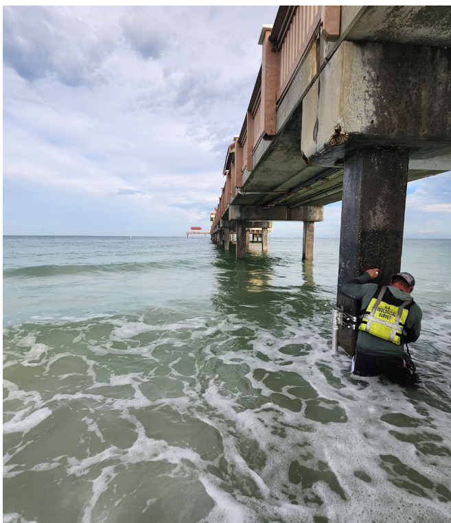
A USGS team member install instruments on a pier in Clearwater Beach, Florida before Hurricane Ian made landfall.
