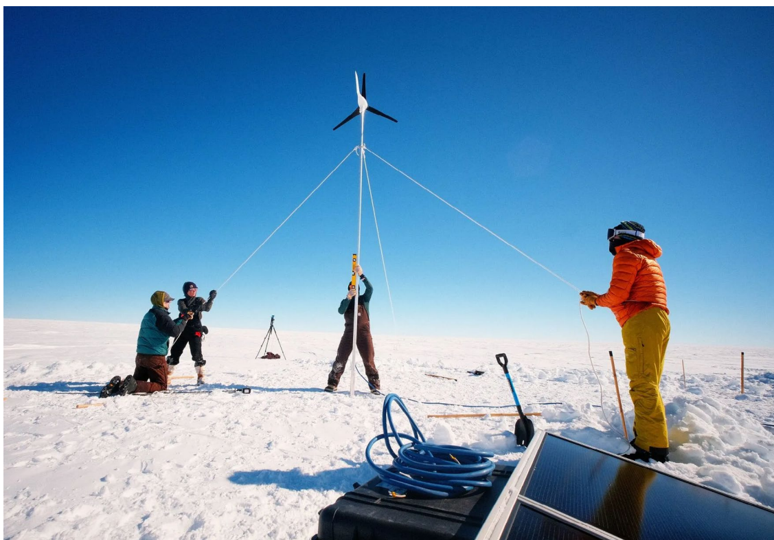
The ICECAPS-MELT field team installs and stabilizes a 14-foot wind turbine. Photo: Michael Gallagher/CIRES
